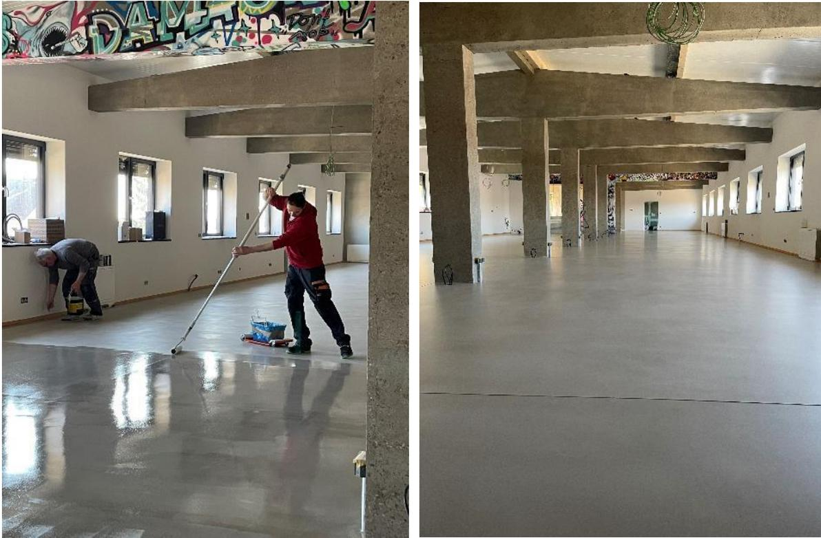
The sealing PCI Zemtec Top gives the directly usable concrete surface a silk matt, optically attractive surface. (Links to the high-resolution photos: [left](#), [right](#))
