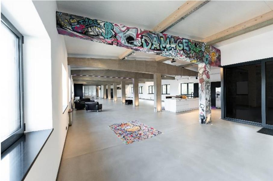
Exposed concrete with PCI Zemtec 1K, sealed with PCI Zemtec Top.
