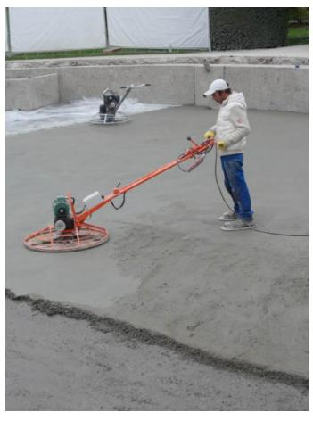
Smooth result: the new screed was carefully evened out. This was helped in the water lily pool by the long, one-hour processing time. Although the visitors to the Wilhelma don't see the smooth finish on the bottom of the pond, it is important for ensuring a permanently intact and sealed substrate.
