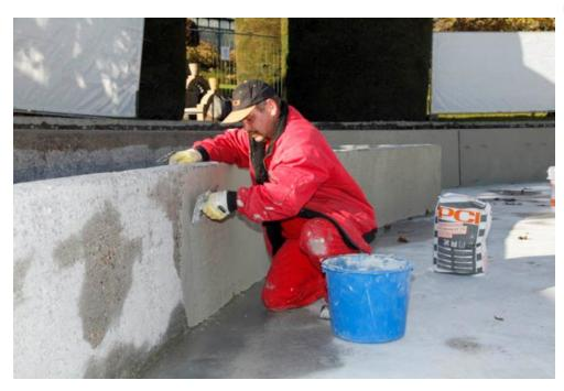
The PCI Nanocret FC fibre-reinforced concrete smoothing compound is particularly easy to handle after the addition of water, as the putty then becomes supple and malleable. Important for application in a water pool: PCI Nanocret FC is water-resistant and weather-resistant. Picture credit: PCI Augsburg GmbH
