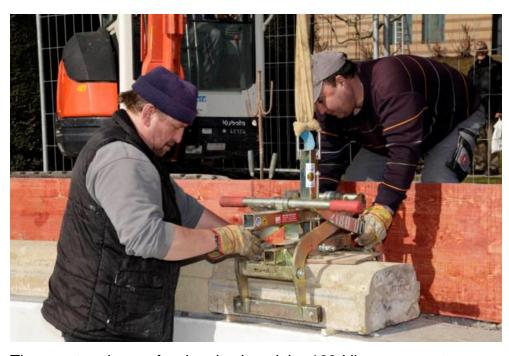
The construction professionals placed the 100-kilogram capstones around the rim of the basin. They wedged the blocks to prevent them from slipping.
