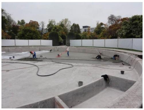
Creating the bonding course, applying the quick-setting screed in a wet-on-wet procedure and smoothing it out – thanks to perfect team work, the construction professionals succeeded in giving the lily pond in the Moorish Garden of the Wilhelma Stuttgart a flawless new surface. The PCI Novoment Z3 binding agent used to coat the screed is ideal for use in the pool. The product is perfectly suited for permanently moist applications and is also particularly temperature resistant.
