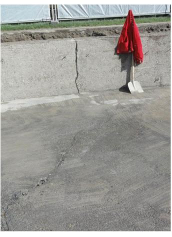
Defects such as cracks and a concave floor which had been scoured away by water over the years were revealed after the pool was emptied.
