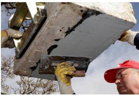
The construction professionals used Durapox NT to replace the capstones on the rim of the water lilly pond basin. First the professionals applied a thin contact layer to the underside of the stones and the rim of the basin. This ensured a professional finish and that the stones keyed well with the substrate.
