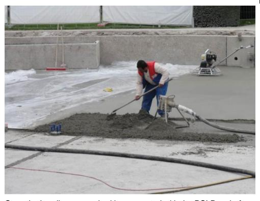
Once the bonding course had been created with the PCI Repahaft mortar bonding agent, the construction professionals laid the new screed on the surface. They worked the screed made of PCI Novoment Z3 fast setting screed cement and screed gravel sand into the bonding course applying a wet-on-wet procedure.
