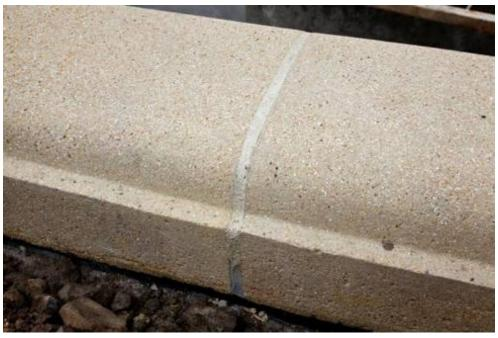
The crowning glory for the water lily pond: the construction professionals grouted the spaces between the blocks of natural stone with PCI Escutan TF. The polyurethane joint compound is ideal for the pond as it is water-tight and resistant to pressurised water. It also does not become brittle over time and is resistant to the weather and root growth. For an overall aesthetic finish, the visible grout was produced by mixing it with a special travertine additive.
