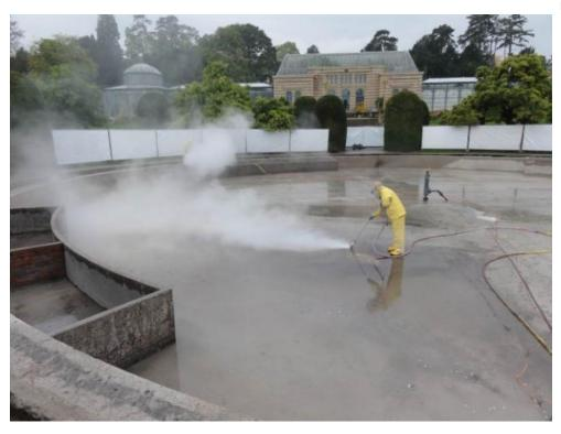
To ensure the subsequent layers bonded well, the concrete surfaces had to be cleaned and roughened by high pressure water jets. This was an effective means of removing loose parts and dirt.
