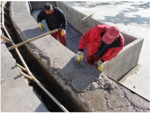
To prevent water leaking from the pool, the construction professionals re-profiled the rim of the basin. The installers used the PCI Bauharz epoxy binder with quartz sand in a ratio of one to ten to prepare the rim of the basin for the listed capstones. PCI Bauharz is waterproof and resistant to weather and frost.
