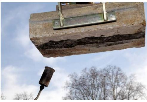
When working with PCI Durapox NT the substrate must be clean, dry, load-bearing and flat. The construction professionals therefore dried out the substrates using a blowtorch.
