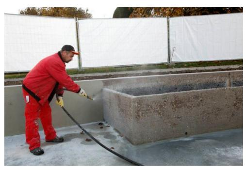
After the substrate had been prepared with the high pressure water jets, the restoration specialists got to work on the inner edge of the pool. The surfaces were first moistened slightly to prevent the three-to four-millimetres thick PCI Nanocret FC fibre-reinforced concrete smoothing compound from drying out.
