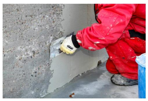
The construction professionals applied PCI Nanocret FC fibrereinforced concrete smoothing compound to the approximately 160square-meter walls of the water lily pond to even out the surface. Picture credit: PCI Augsburg GmbH
