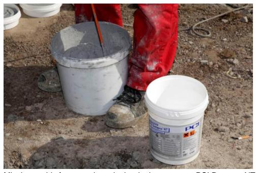
Mix thoroughly for a good result: the dual-component PCI Durapox NT reaction resin binder must be handled exactly according to the instructions. The base and hardener component are therefore blended intensively in the specified mixing ratio for at least three minutes, until a uniform colour is achieved. The construction professional then fills a sufficiently large bucket with the mixed binder and mixes in quartz sand.
