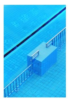
The tiles were laid and grouted using PCI Durapox NT plus chemical-resistant, water-impermeable adhesive. The adhesive sets without cracks and cures without shrinkage – for joint widths from 2 to 20 mm.
