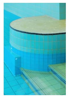
The ceramic tiling in the swimming pool itself, with an area of about 700 m<sup>2</sup>, was laid and grouted using the twocomponent reaction resin adhesive and grouting compound.
