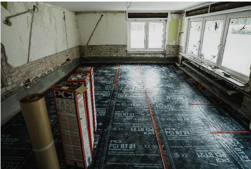
Modern waterproofing technology with the cold-applied, self-adhesive waterproofing membrane PCI BT 21 which is easy and quick to apply. ( Link to high-resolution photo )
