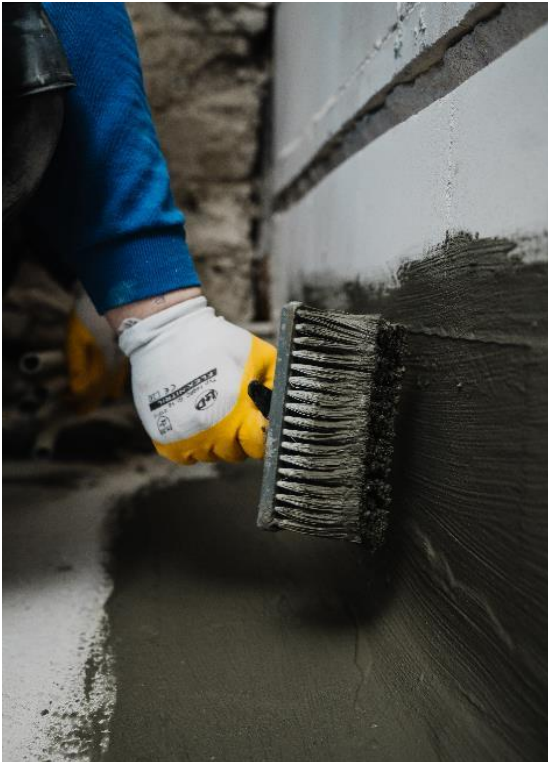
The mineral waterproofing slurry PCI Barraseal protects against moisture penetration. ( Link to high-resolution photo )
