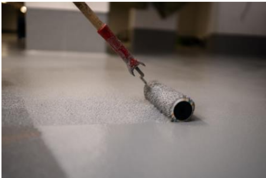
Rolling the top layer PCI Apoten OS TC (link to the high-resolution Photo )
