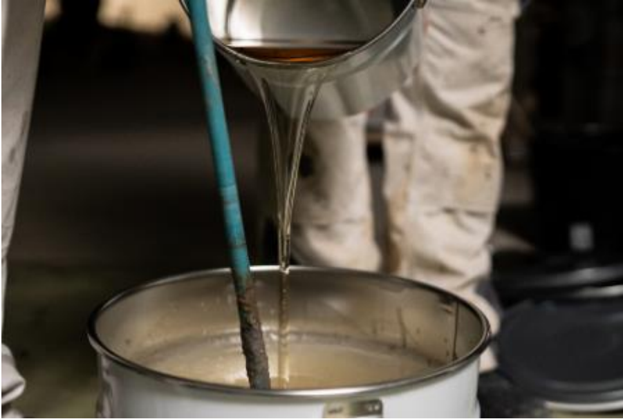
PCI Apoten OS P consists of the basic component A and the hardener component B which is added. (Link to the high-resolution Photo )
