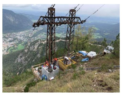
From corrosion protection to grouting, only PCI building materials were used. PCI specialist advisor Marcus Donhauser and PCI service technician Jürgen Linke were on site.
