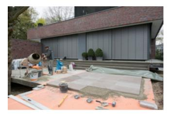
The Pavifix DM is mixed with water in a free-fall mixer before being applied to the single grain mortar membrane in a 5 cm thick layer. **Picture credit:** PCI Augsburg GmbH
