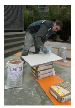
Step by step, the patio takes shape. In order to ensure optimum adhesion, the tilers apply Carraflott NT to the back of the natural stone with 6 mm toothed trowel. The slab is then turned over and tapped into place in the fresh Pavifix DM mono grain screed.
