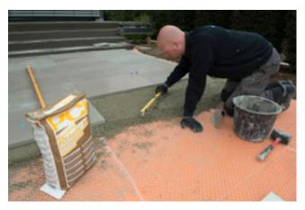
Accuracy comes first: once a 5 cm thick layer of PCI Pavifix DM has been applied, Benjamin Wyß checks the evenness of the surface. **Picture credit:** PCI Augsburg GmbH
