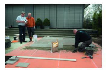
A Schlüter single grain mortar membrane is laid before a 5 cm layer of PCI Pavifix DM drain and screed mortar is applied. **Picture credit:** PCI Augsburg GmbH
