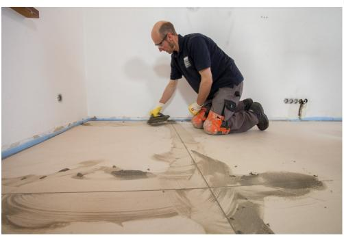
The fully vitrified tiles were grouted using PCI Flexfug.
