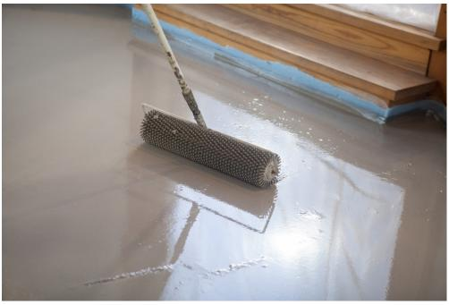
PCI Periplan Extra is distributed with a skid leveller and then levelled and aerated using a spiked roller.
