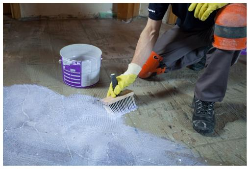
The entire surface was prepared for laying large tiles using PCI Gisogrund 404 primer.
