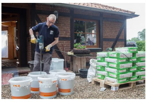
Jens Pomplun used the fibre-reinforced special levelling compound PCI Periplan Extra for levelling the screed.
