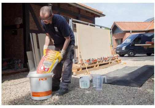
The master tiler mixed PCI Rapidflott flowable tile adhesive with the polymer-modified additive PCI Lastoflex.
