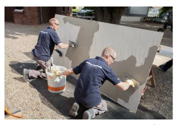
To ensure laying with virtually no voids, PCI Rapidflott was applied both to the substrate and to the back of the tile.
