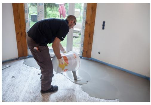
PCI Periplan Extra special levelling compound flows easily and can be processed without any problems.
