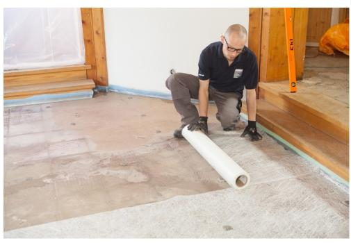
PCI Armiermatte GFM glass fibre reinforcement was used to reinforce the levelling compound.
