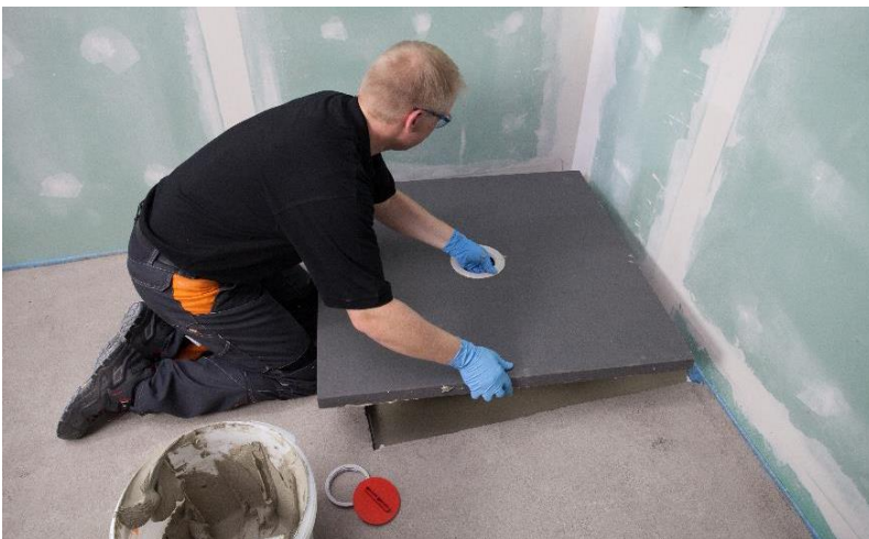
Level-entry showers - easily installed with PCI PowerBoard Waterline (link to high-resolution Photo )
