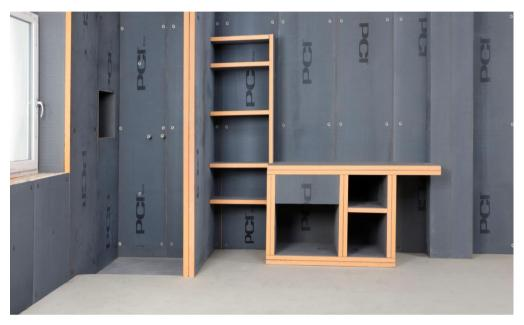
PCI PowerBoard is the new supporting element system of PCI Augsburg GmbH for interior construction and renovation – with perfectly fitting, sturdy supporting elements for level substrates and angle elements for corners and pipe cladding.
