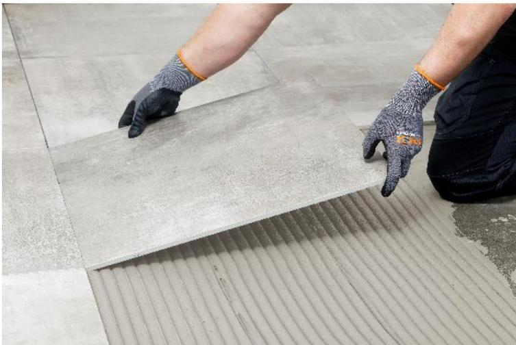
*The new PCI Nanorapid fast-setting adhesive speeds up work processes and increases application convenience* ([Link](#) to high-resolution photo)
