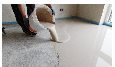
The new PCI Periplan Flow leveling compound with exceptional flow properties (Link to high-resolution Photo)
