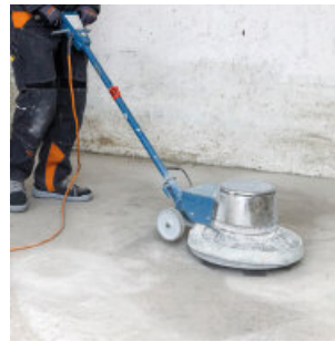
Grinding the floor
