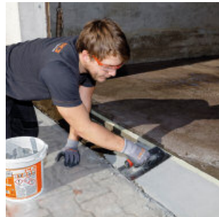
Finally, smooth the mortar
