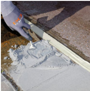
Apply PCI Aposan® reaction resin mortar to the fresh primer
