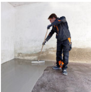
Distribution of leveling compound
