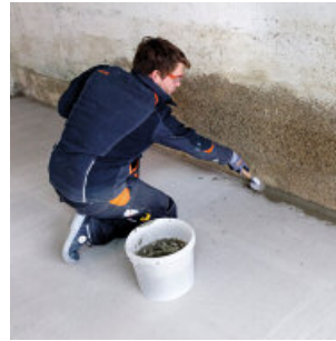
Installation of concave moulding
