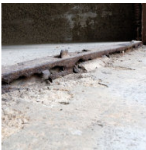
Damaged screed rail
