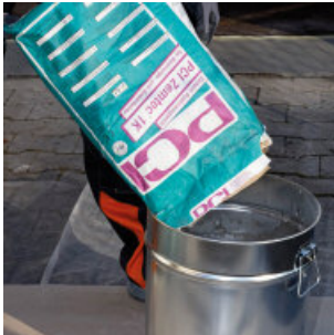
Preparation of the floor leveling compound
