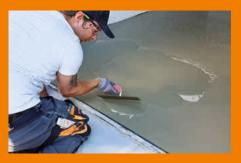
Despite its liquid consistency, PCI Zemtec Outdoor can be easily applied to drains and edges without sagging.
