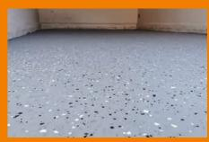
Optically enhanced with color chips and protected with PCI Zemtec Protect, PCI Zemtec Outdoor creates a floor that can be used directly in outdoor areas exposed to weather conditions or in indoor areas exposed to wetness.
