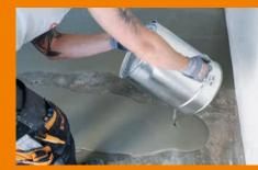
The directly usable mineral coating is poured out and can be spread without effort.
