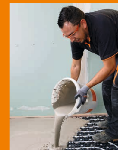
The fiber-reinforced leveling compounds in the PCI Periplan family are the ideal choice for floor leveling over underfloor heating systems.
