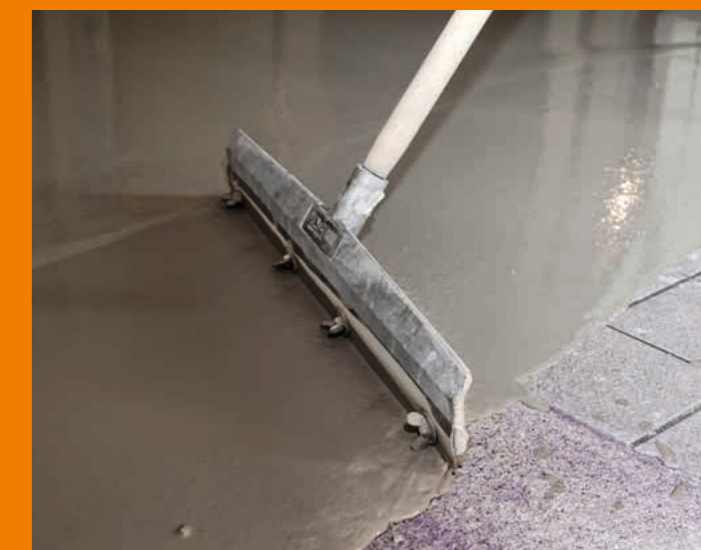
Using a pin or skid leveler, the leveling compounds in the PCI Periplan family can be distributed conveniently from a standing position.
