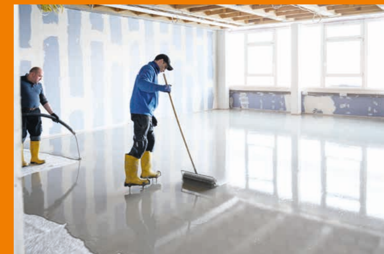
All the leveling compounds in the PCI Periplan family can also be applied using a pump.
